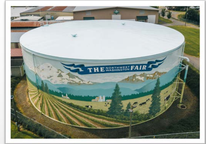
3MG Tank Roof Repainted
